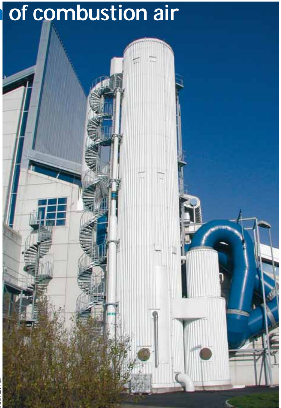
Scrubber tower for cooling of flue gas and humidification of combustion air at the wood-fired Allö plant in Kristianstad, Sweden.
