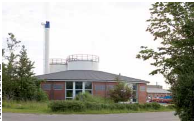
The existing natural gas CHP-plant. One of its engines will now be converted to run on gasification gas.
