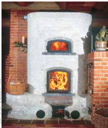
The masonry stove is a low-tech but effective method of reducing particle emission.
