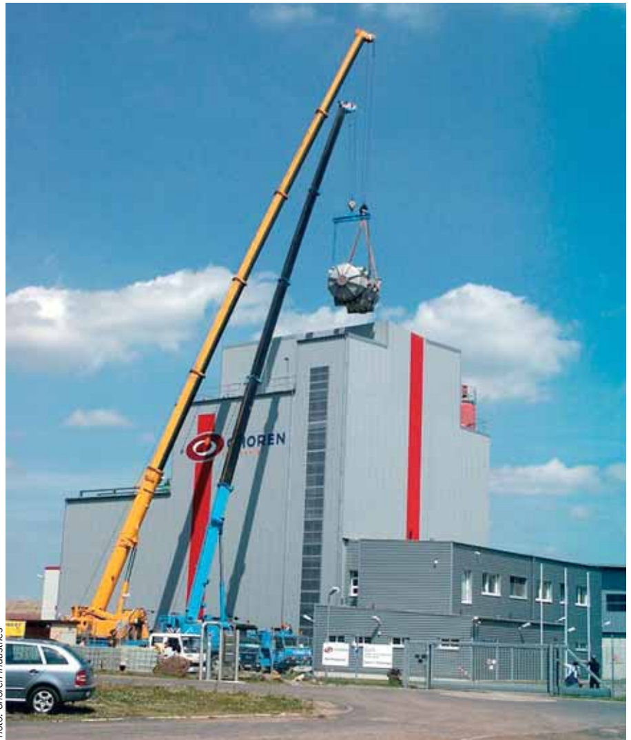
Installation of low-temperature gasifier on the plant in Freiberg.
